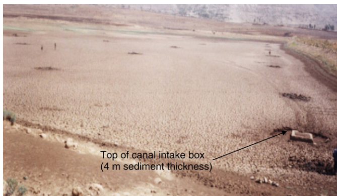
Fig. 2. Adikenafiz reservoir. The top of the inlet canal is clogged due to excessive sediment deposition and is shown cleared from sediment.
